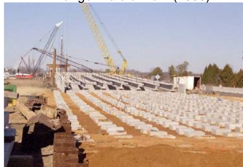
Lord Delaware bridge, Virginia - U.S.A.(Hoppe e Hite, 2006)
